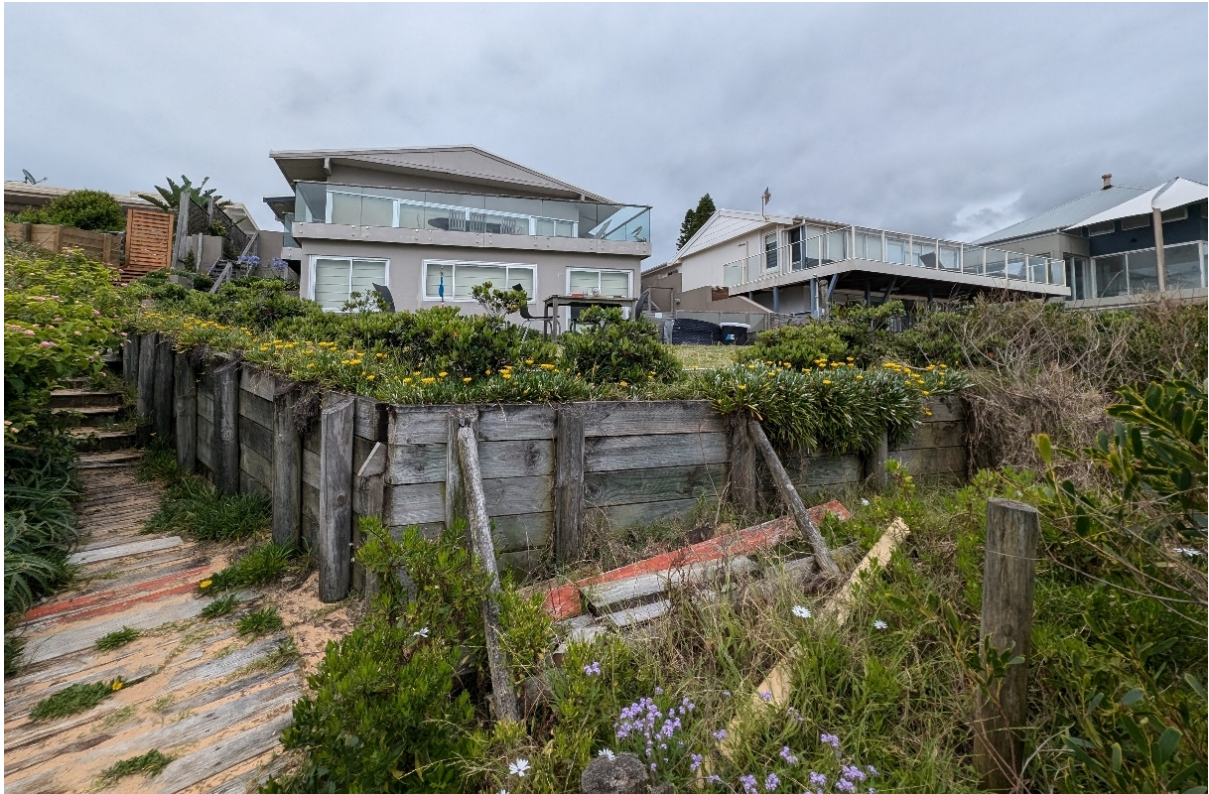
Figure 8 – Ad hoc protection works to rear of Calais Road property
