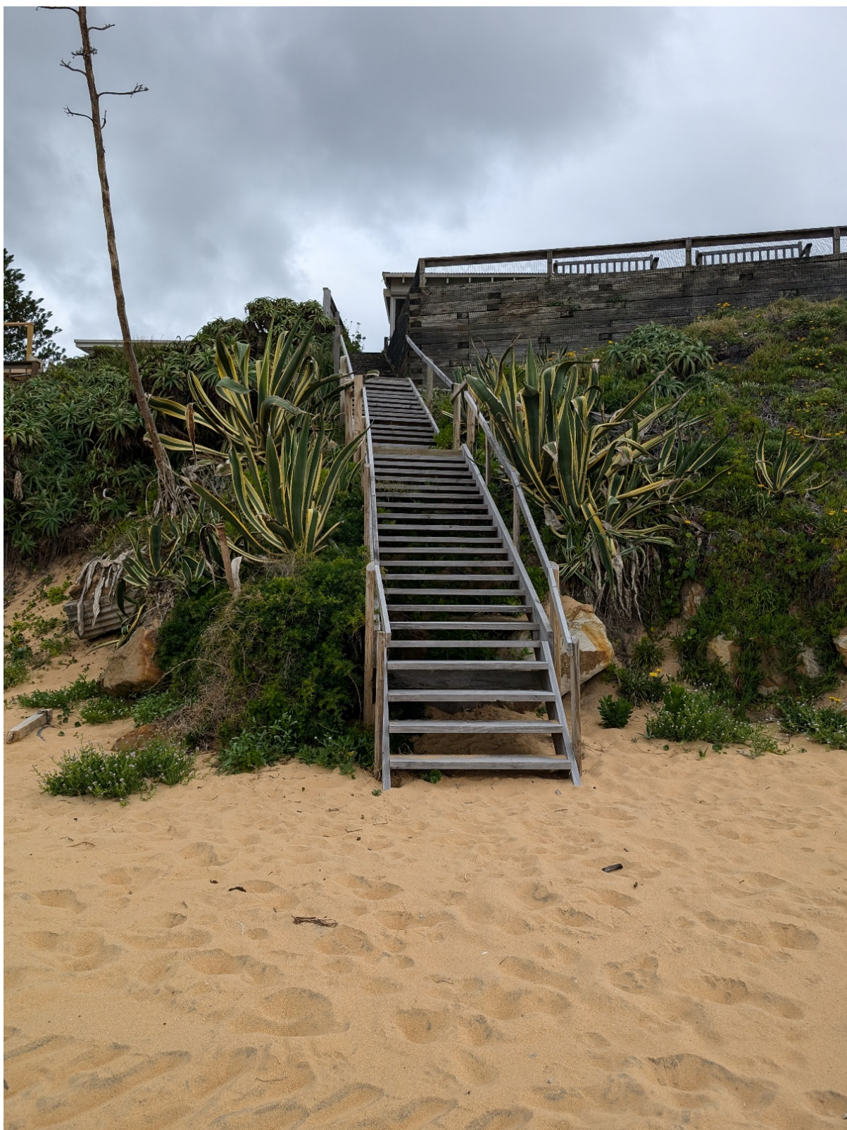
Figure 7 – Ad hoc protection works and access stairs to rear of Calais Road property
